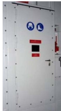
A properly closed door
