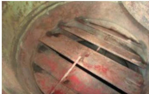
PSC detainable deficiency
